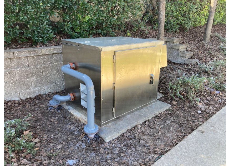
East Branch Pkwy @ Arlington Rd
