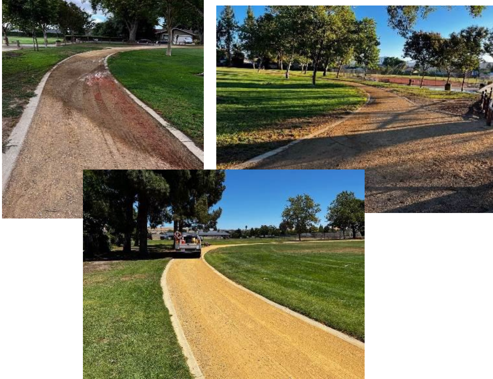
Boone Acres Park Track Renovation
