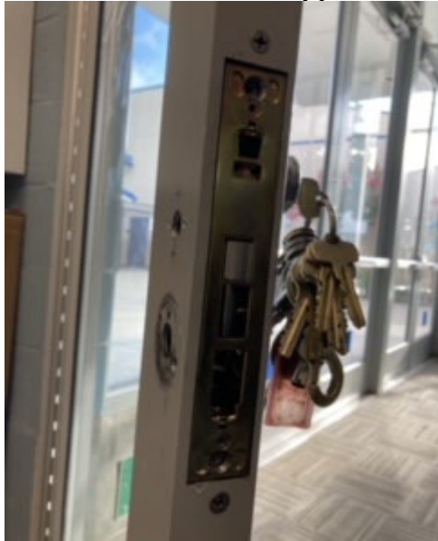
Door Hardware Replacement
